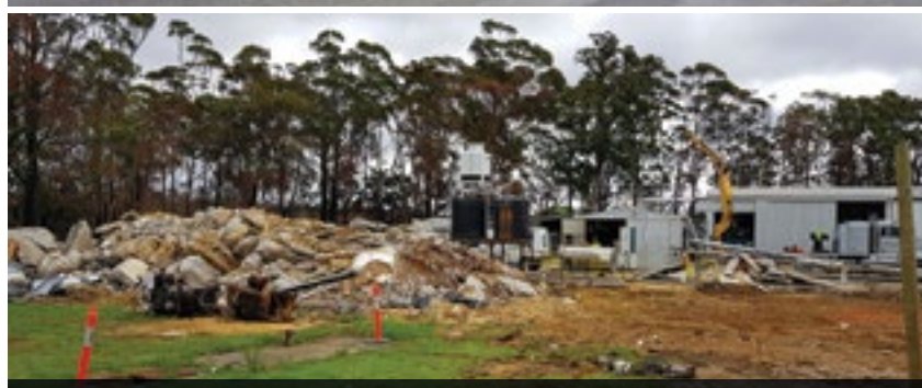
Destroyed by fire: AFCOL abalone processing plant before and after the fire – Image supplied
