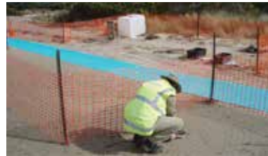
An onsite decontamination station was practiced
